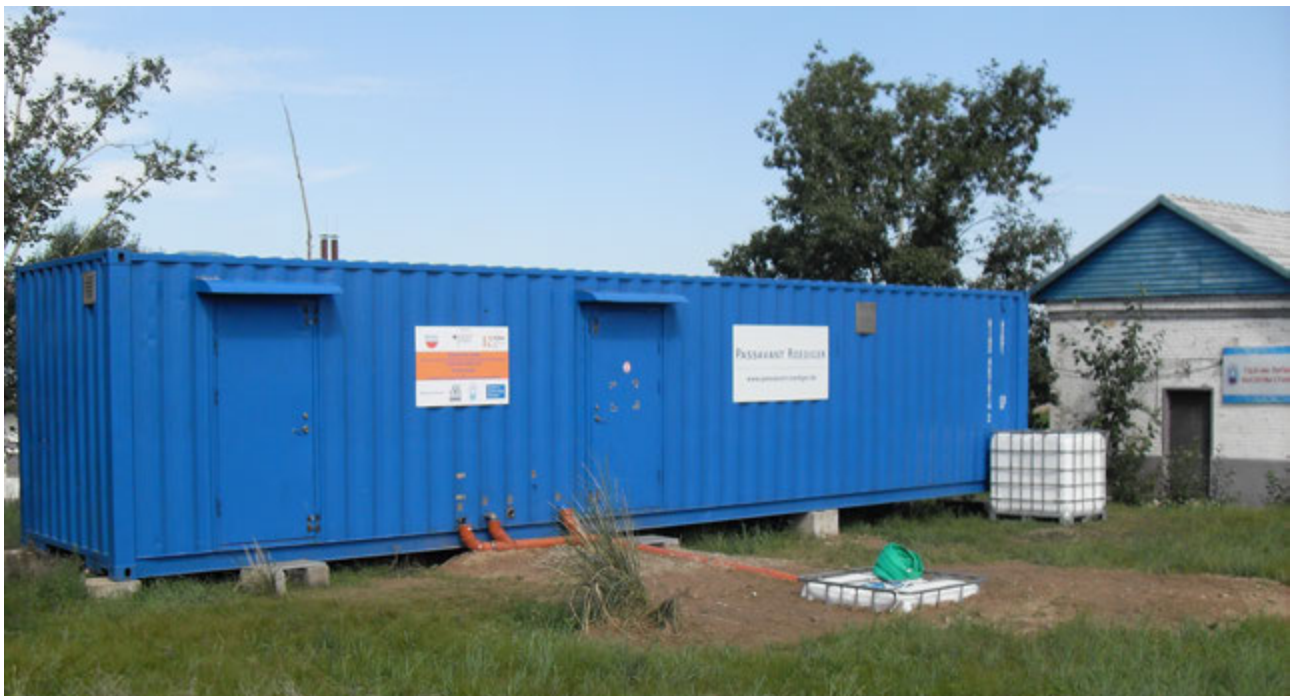
Fig. 1: Biogas pilot plant installed in a 40 ft shipping container (location: WWTP Darkhan)
