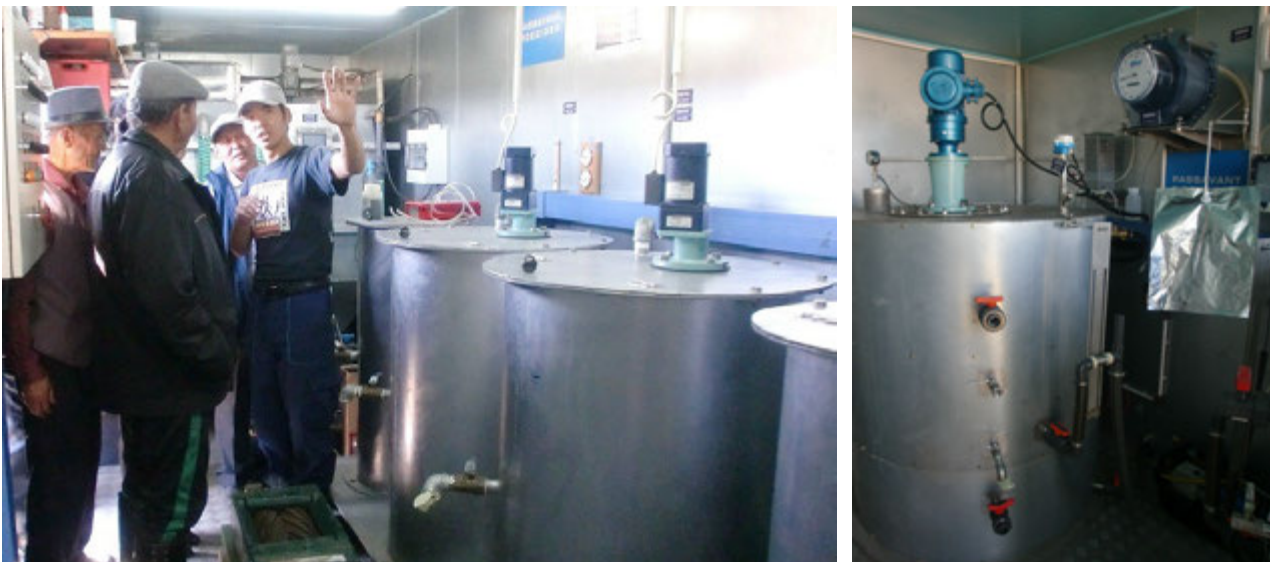
Fig. 2: Local operator of the plant explains storage & mixing section to inhabitants of Darkhan (left); digester (right)
