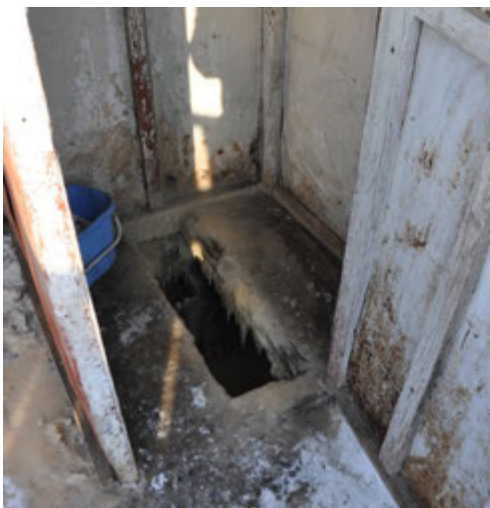
Fig. 3 (left): Old latrine: no user comfort, very unhygienic, contaminating the environment and dangerous to use in wintertime when the ground is frozen.
